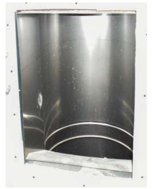
Shaft and brake lane
